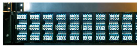
2U chassis can accept up to 12 modules offering 288 fibres (144 per 1U) on a standard LC quad adaptor.
